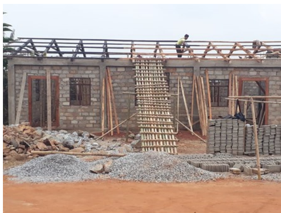
The Edmund Rice Hall getting constructed in collaboration with people
